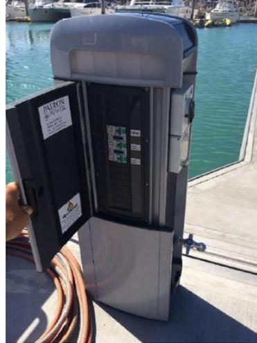
Both are able to supply all your power needs safely. As per Australian Electrical Safety Standards, all power supplied by the pedestals have 2 separate safety switches installed which can pick up different possible faults. BOTH must be on for your power to be active. These devices are:
